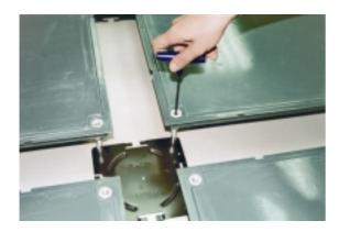
Leveling adjustment: Use 4 mm hex key wrench and adjust height from top.
